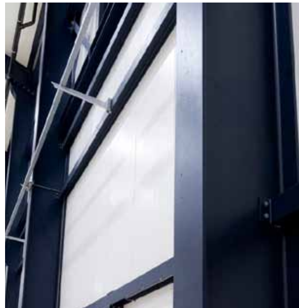
Detail of steelwork, Rotterdam Airport, Netherlands
